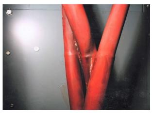
Figure 2 Phase to phase PD caused by poor installation
