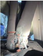
Figure 4 11kV RMU Termination Failure
