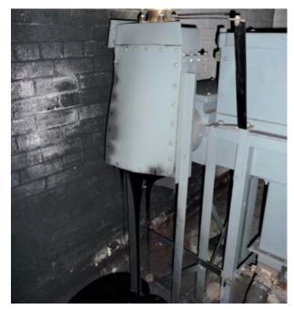
Figure 1 Failed bitumen filled cable box
